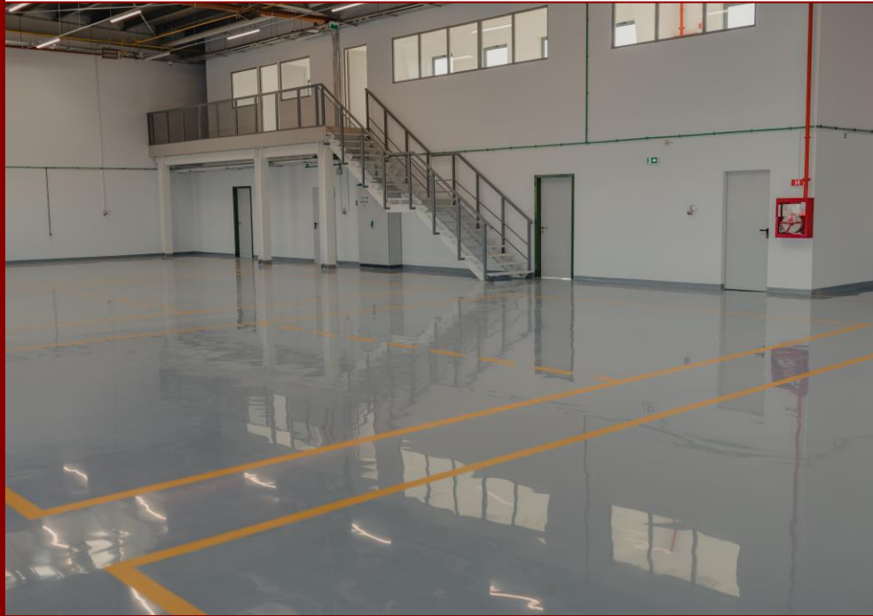
Floor Finishing – PU Flooring
